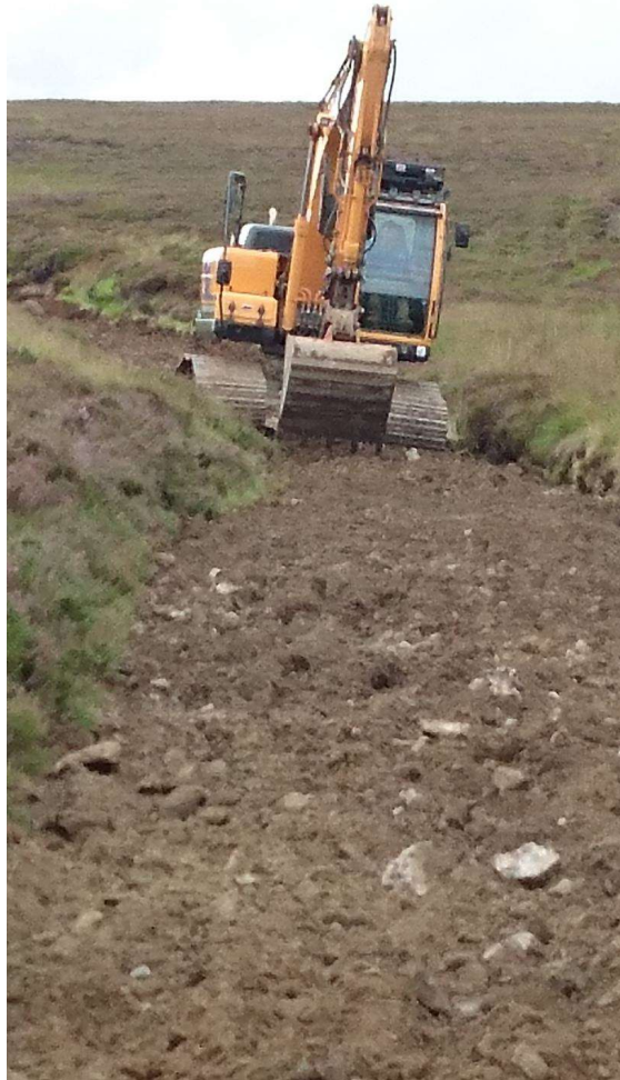
Maintenance/repair – or more substantial upgrade requiring Prior Notification? Glen Clova, summer 2017.
