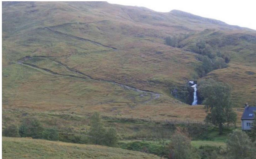
Long-standing track, Iron Lodge, Glen Elchaig, Wester Ross – photographed October 2015. Images on www.geograph.org.uk/photo/5193548 show this to be more than 25 years' old; note the short cut that has been created.
