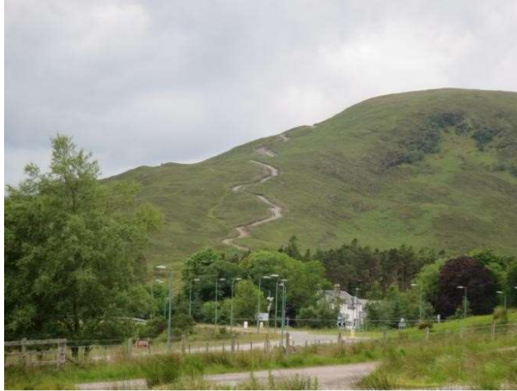
Track at Ledgowan, Achnasheen; photographed June 2017; more than five years after construction it remains highly intrusive in this sensitive landscape
